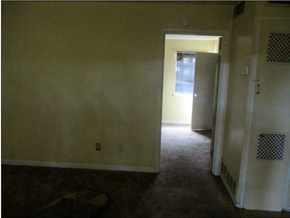
Typical interior view within one of the vacant units (to be renovated)
