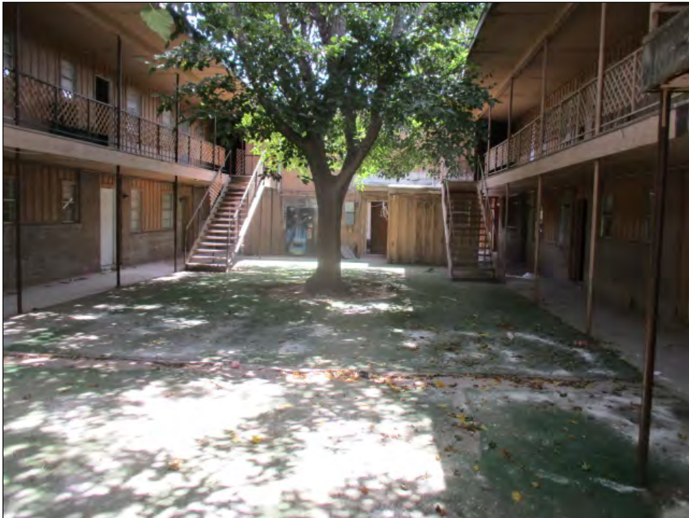
Typical view of central courtyard area
