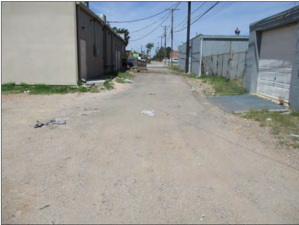
Looking west along the 20-foot-wide dedicated alley
